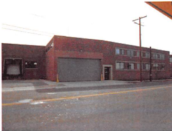
Lease 5 V Street Industrial Warehouse
