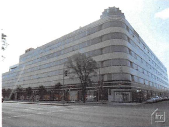
Lease 1 Hecht Warehouse District, Tower I and II
