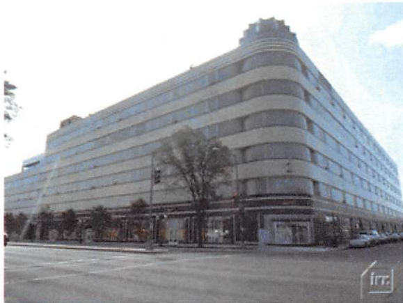
Lease 3 Hecht Warehouse District, Tower I and II
