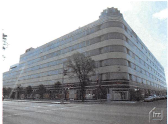
Lease 4 Hecht Warehouse District, Tower I and II
